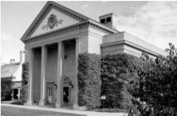
George Eastman House, the Dryden Theatre. Courtesy of George Eastman House
