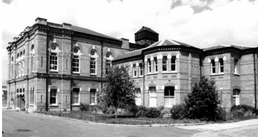
The Cinema Museum, the Master's House, Kennington, London, formerly the administration block of the Lambeth Workhouse.
